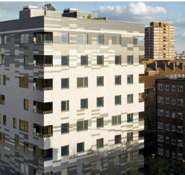
Murray Grove Residential Building, UK
