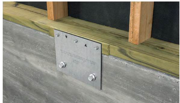
Reinforcement of the connection with the foundation
